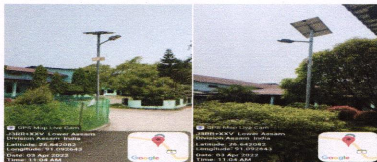
Figure 8: Solar light inside the college campus
